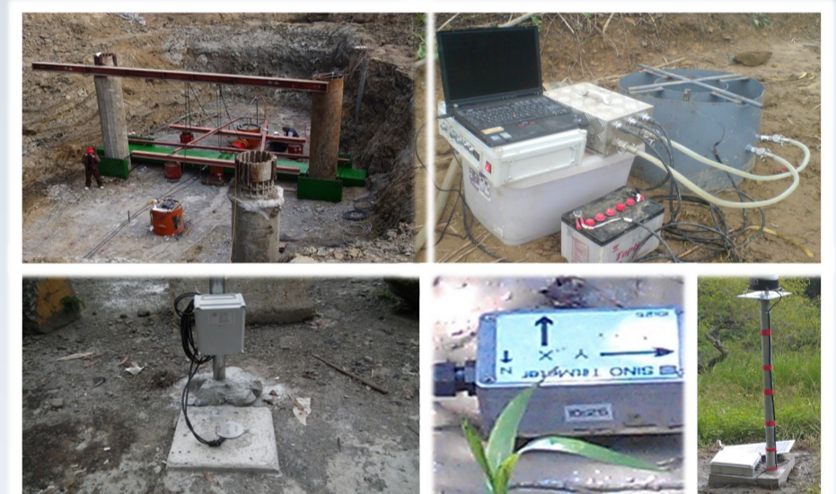
▲ Pile Load Test
