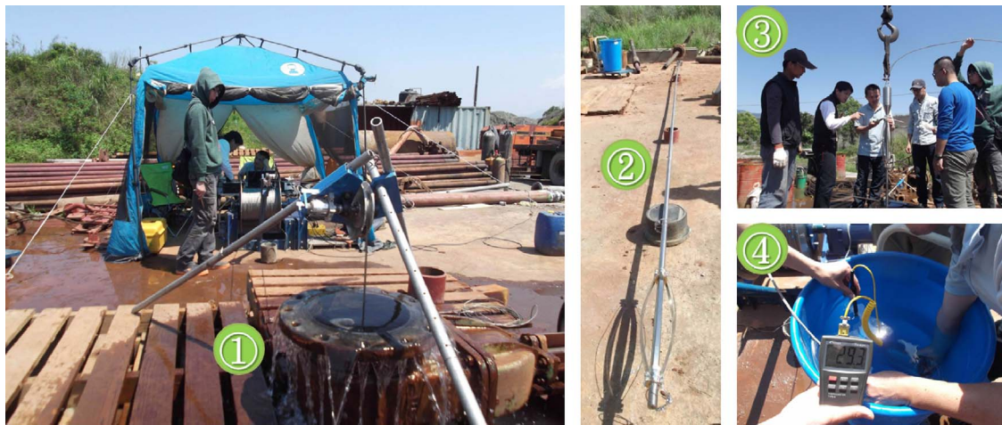
Fig. 5. Site Operations in JY-01 Test Well.
