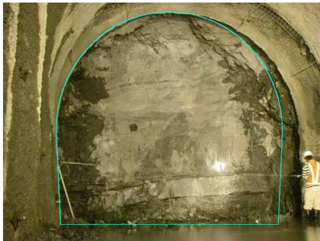
Figure 4 – Typical rock mass conditions for the case tunnel
