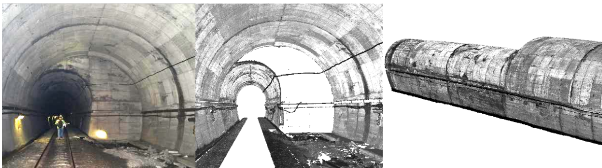
(a)現場照片 (b)隧道雷射掃描 3D 點雲 (c)雷射掃描 3D 影像外視圖
