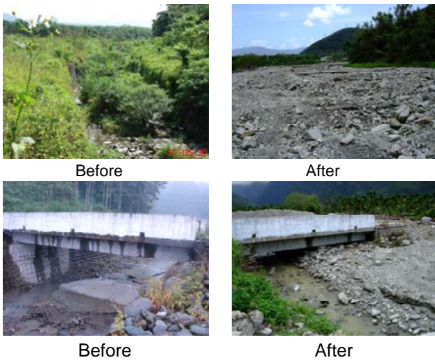
Fig. 10. Before and after photos of Typhoon Fenghung in the Hualien A124 creek.
