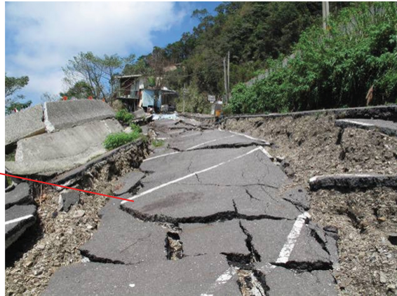
圖 16 莫拉克颱風藤枝地區崩滑破壞情形 Fig.16 Teng-Zhi area collapsed during Morakot typhoon.
